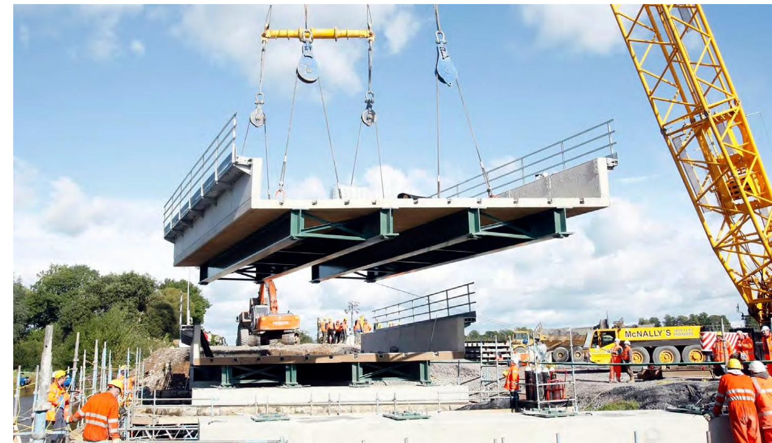
1 Road Bridge Reconstruction
