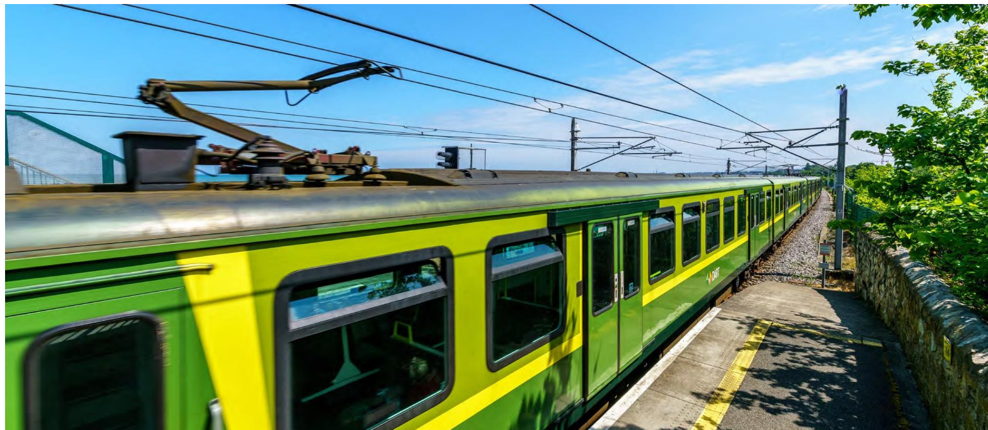
20km of Overhead Electrification & 6 New Substations
