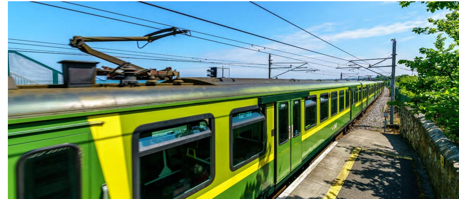
37km of Overhead Electrification & 8 New Substations
